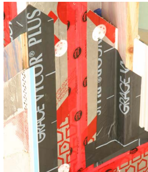
All corners and joints are taped for optimal air leakage control
