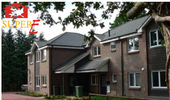
Downland Housing Association set a new performance standard for social housing with this SuperE building from DAC
