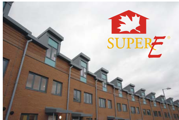
Southern Housing Group's Lewis Gardens is a DAC SuperE™ project.
